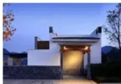
Household Energy Storage
